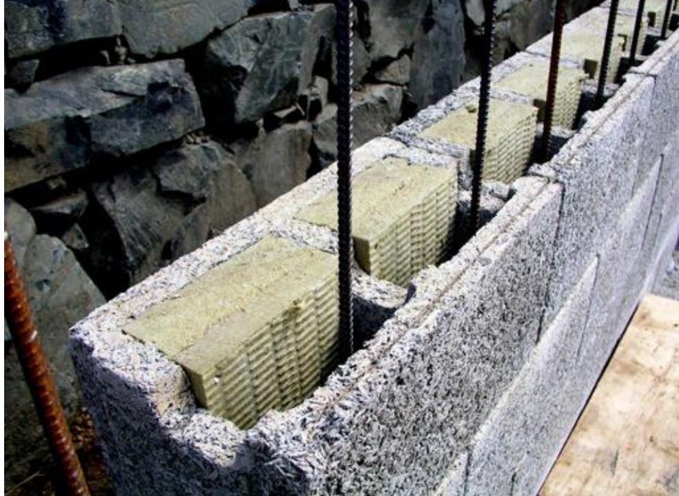
Clockwise from top left: schematic of dining area; blocks of Durisol, a proprietary material made of cement-bonded recycled-wood fiber that creates a breathable wall; schematic rear of home. ILLUSTRATIONS COURTESY TERRACEWOOD.CA.
